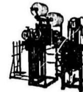
Right: PETERS SENIOR CARTON FOLDING AND CLOSING MACHINE — A fully automatic machine which closes cartons at speeds up to 50-60 per minute. This machine operates in coordination with your packaging line. JUNIOR Model available to handle smaller production programs.
